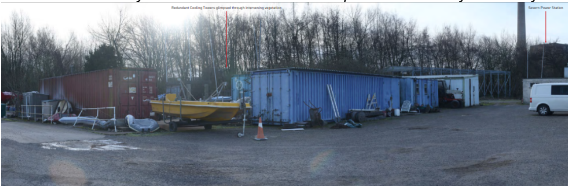
Taken from Newport Uskmouth Sailing Club car park, looking south-west towards the site – existing cooling towers barely evident due to distance and intervening features (extracted from LVIA)
